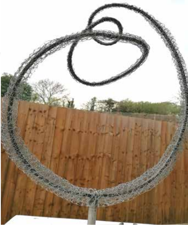
Adding chicken wire for plaster
